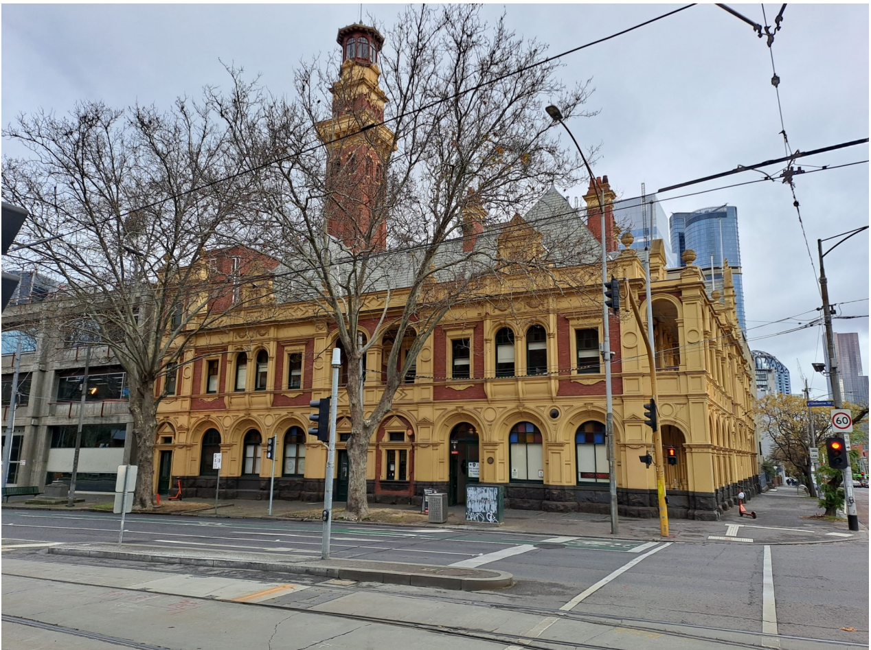
Old Eastern Hill Fire Station—Our November Meeting Place.
